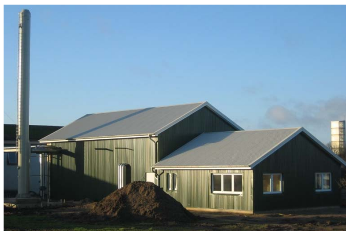
co-generation plant- and office building
