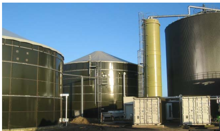
hydrolysis, post digester, desulphurisation, digester
